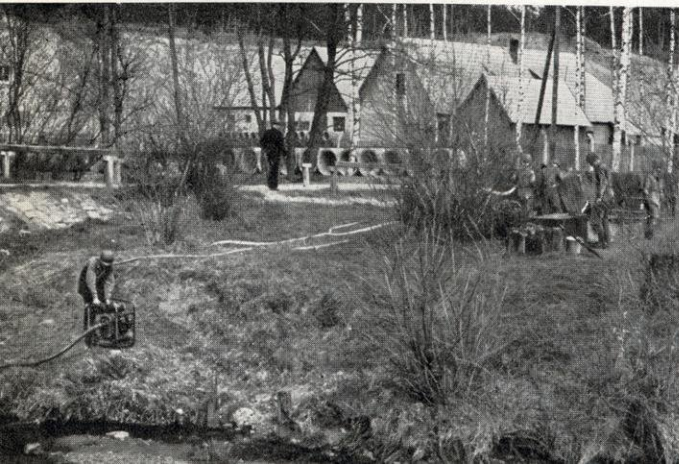
Water is pumped from running stream, filtered, purified and put into vats for use of 2nd Armored Cavalry.
