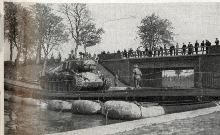
Sherman tank crosses the 1st Combat Engineer Bn's bridge at Neu-markt, during advance on Bamberg. Bridge supports 50 tons.
