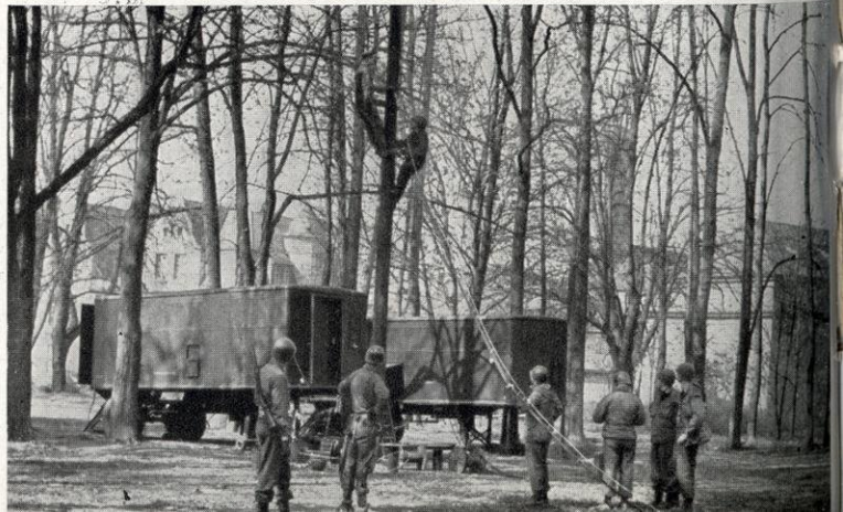
Wiremen of the 776 Signal Service Company set up wires for telephone and teletype operations at Stein Castle.
