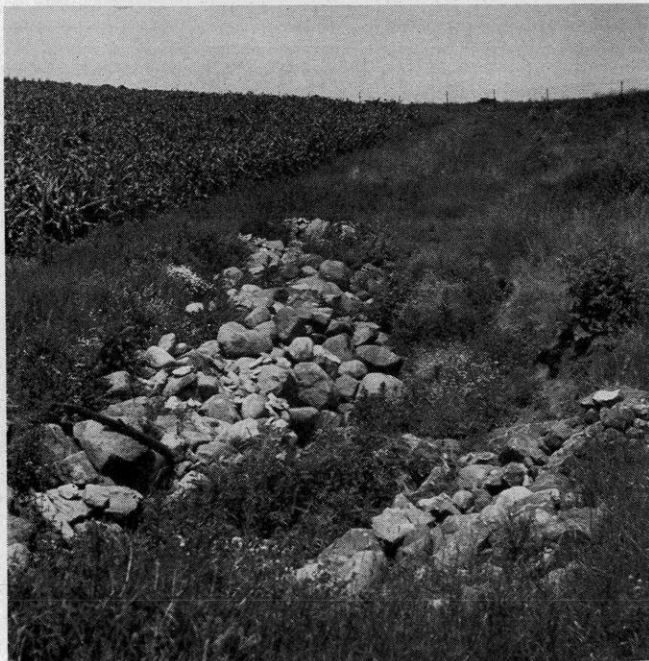
EROSION CONTROL, OLD STYLE
