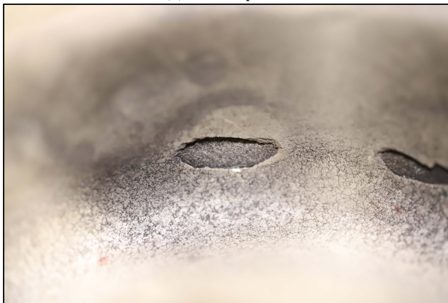
(b) View close to a delamination spot
