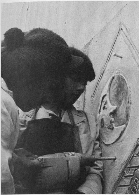
Two students work together to drill holes through the tile and the concrete wall in order to bolt the tile in place along one wall of the interior courtyard, detail. Photo courtesy of Nan Park and Joe Perretti.
