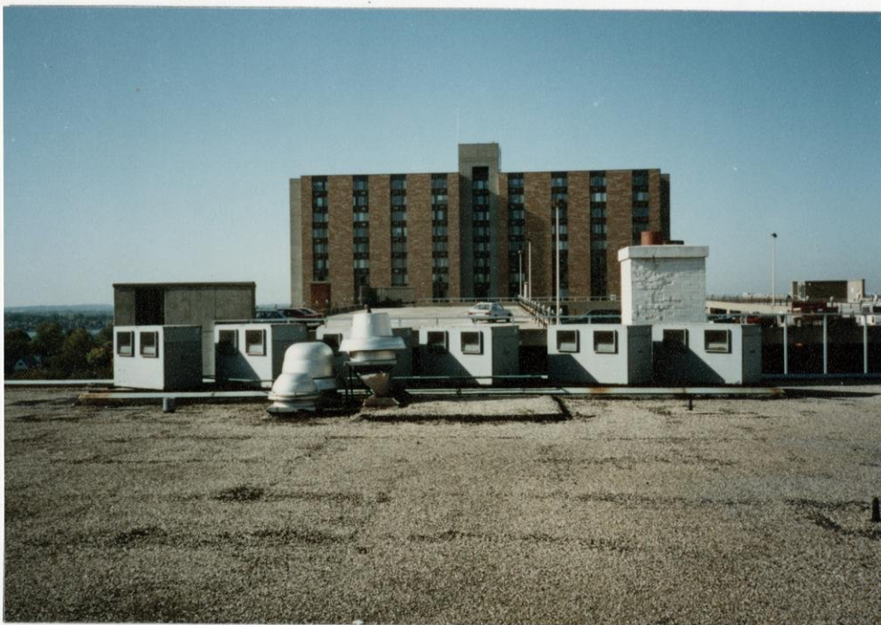
View of roof showing roof-top compressors.
