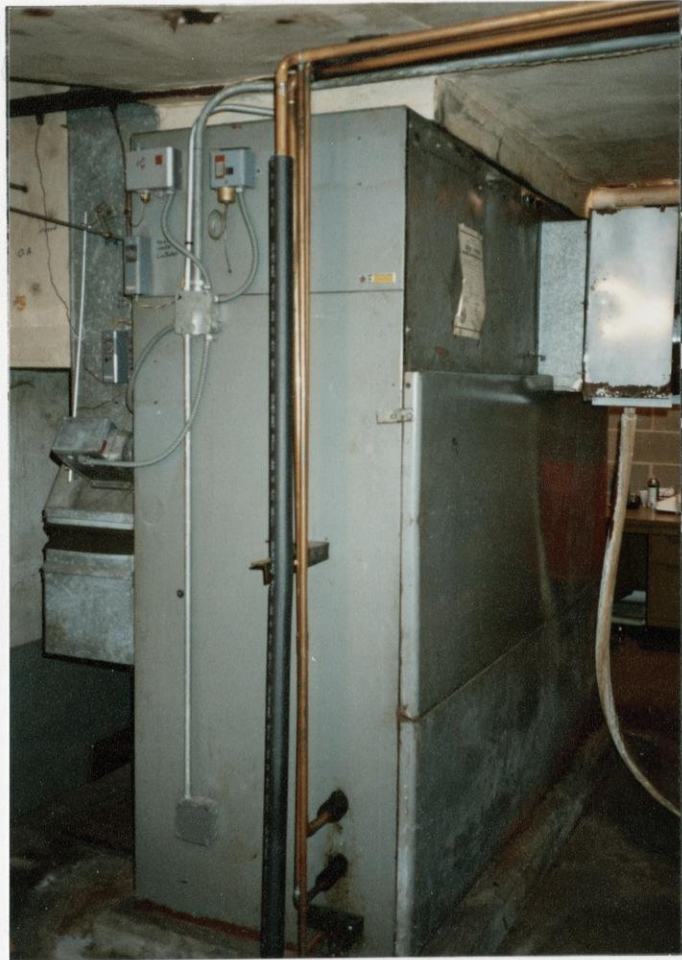
View of typical air conditioning/air handling unit.
