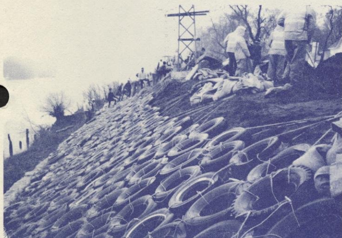
Eau Claire—Dike work. Old tires were used in profusion to strengthen the Forest St. dike on the Chippewa River. Such actions minimized the damage from flooding this spring.
