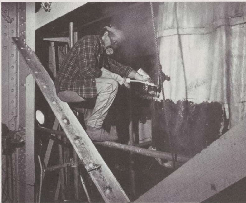
With a cryogenic process first used here, a worker blasts away old paint from inside the Statue of Liberty. The black area is the coal tar undercoat; above it is paint yet to be removed.
