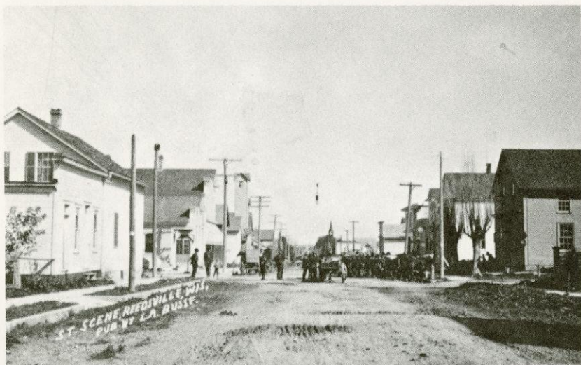
Scene looking east on Manitowoc Street: Building on left was a tavern now moved and the home of Charles C. Vondrachek. Next building now Kabats Tavern. Building on right now Savages Tavern.
