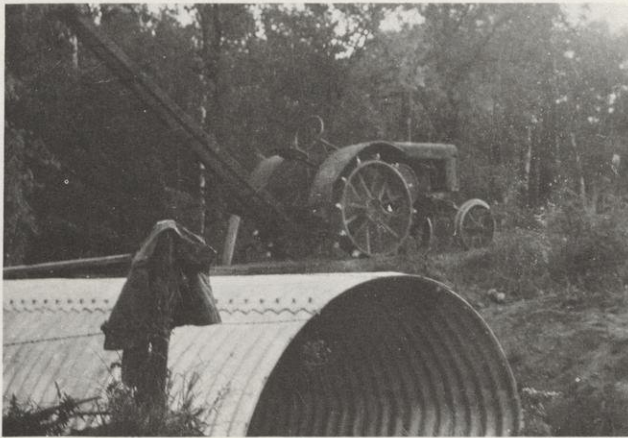
Crew setting street culvert together.
