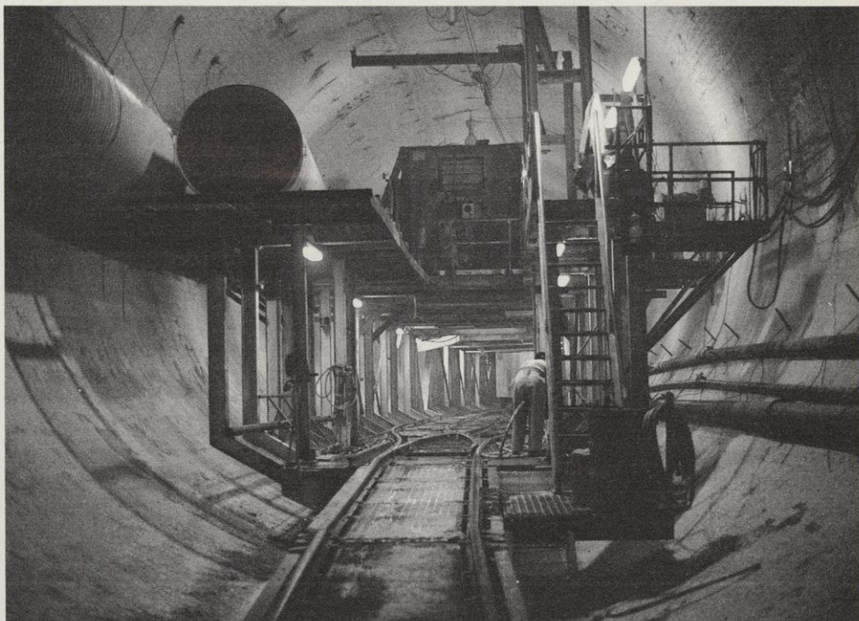
When rain and snow fall hard and heavy, 17 miles of tunnels under Milwaukee will hold sewage and storm water. During drier weather, this liquid will be pumped to the surface for treatment.
