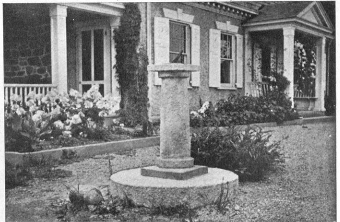
SOME VERY ROUGH STUCCO IS SHOWN ON THE WALL OF THIS HOUSE AND IN THE FOREGROUND A CONCRETE SUNDIAL — HOME-MADE — USING AN OLD MILLSTONE COVERED WITH STUCCO FOR A BASE.
