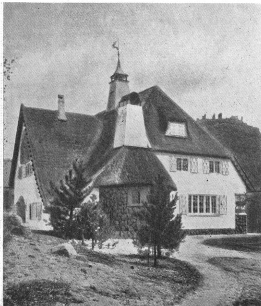
ONE CORNER OF THE BUILDING SHOWN ON PAGE 548, SHOWING THE USE OF STONE IN THE FOUNDATION AND CIRCULAR WALL.
