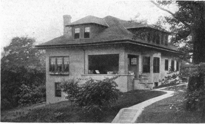
THIS HOUSE, 30 FEET BY 48 FEET IN PLAN, BUILT OF CONCRETE AND FRAME, IS IN A SUBURB OF PITTSBURGH. IT WAS DESIGNED AND BUILT BY W. H. PARRISH FOR $4,600.
