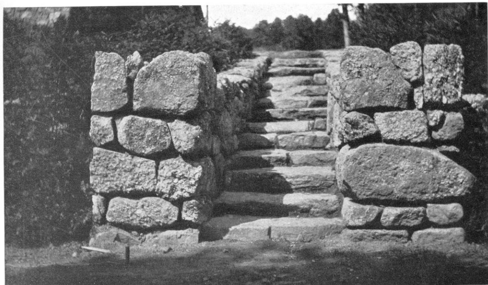
THE LOG HOUSE AT CRAFTSMAN FARMS, SHOWING THE BEGINNING OF THE PLANTING OF THE GARDEN AND THE BUILDING OF THE WALLS. A DETAIL VIEW OF THE ROUGH STONE STEPS FOR THE GARDEN WALL: THE STONE PILLARS ARE BUILT HOLLOW SO THAT LATER ON THEY MAY BE FILLED WITH EARTH AND PLANTED WITH FLOWERS AND VINES.
