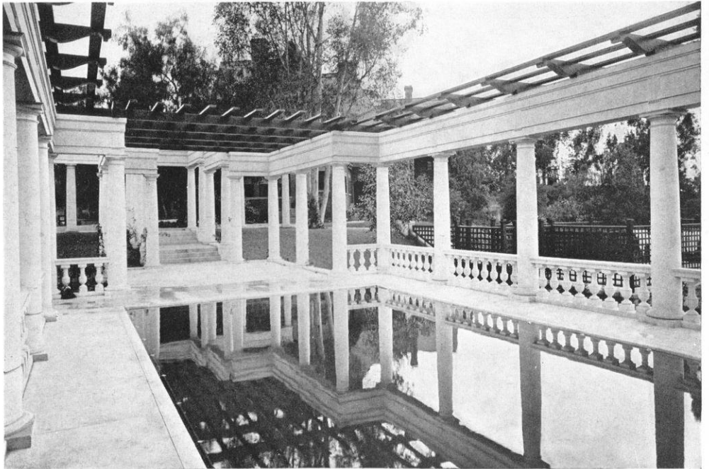
TWO PHOTOGRAPHS OF A SMALL POOL IN A FORMAL GARDEN: THIS POOL IS TEN FEET WIDE AND TWENTY FEET LONG AND GRADUATES IN DEPTH FROM THREE FEET SIX INCHES TO SEVEN FEET: THE WASTE WATER FROM THIS POOL IS USED FOR IRRIGATING THE GARDEN.
