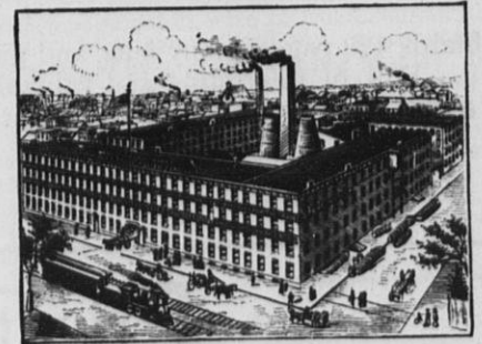
(View of Works.)
