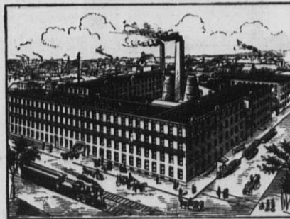
(View of Works.)
