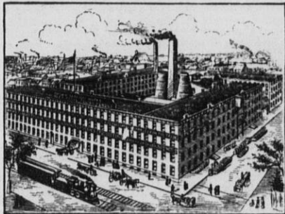
(View of Works.)
