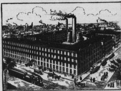
(View of Works.)
