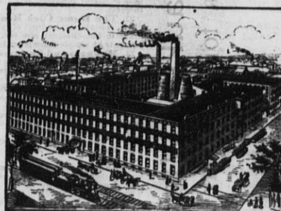
(View of Works.)
