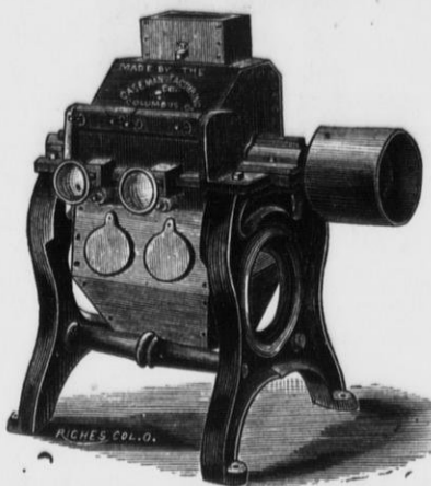
Single Break Machine, capacity 5 to 60 bushels per hour.
