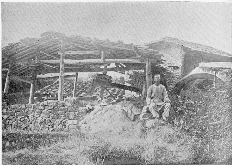
Mill for pounding the rock
