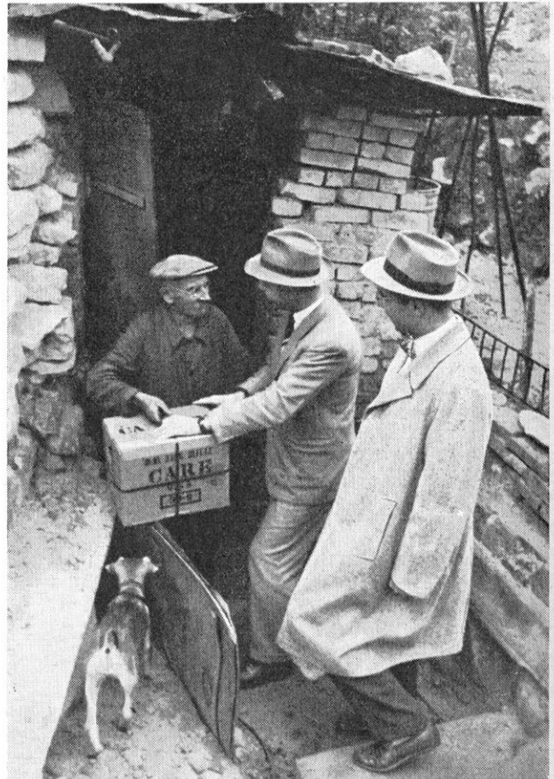
A blind German worker, living in the basement of a war-wrecked building, receives a food package from Frankfurt CARE workers. At right is James Stanley, member of the CARE Mission and the author of this article.
