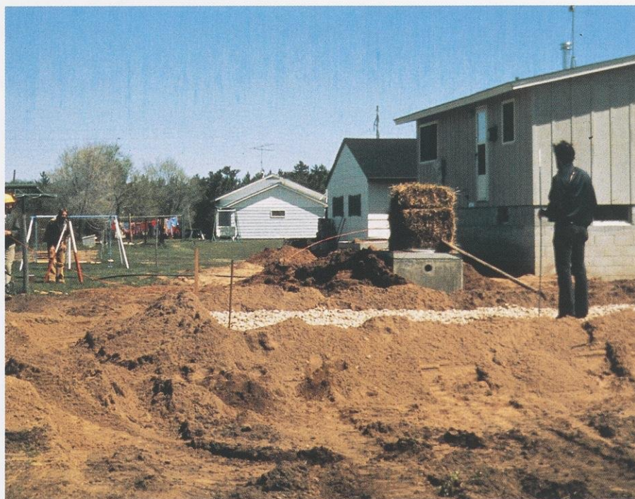
Installing a sewage drainage field.
