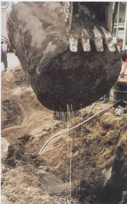
An aggressive program aims to locate, replace or remove buried tanks that can leak stored fuels. Few tanks leak this badly, but even small amounts of gasoline make water unfit for use in residences, businesses and for animals. Cleanups are expensive.
