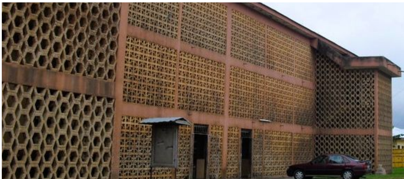
FIGURE 5.3: The walled-off exterior of the Kwahu South District Assembly
