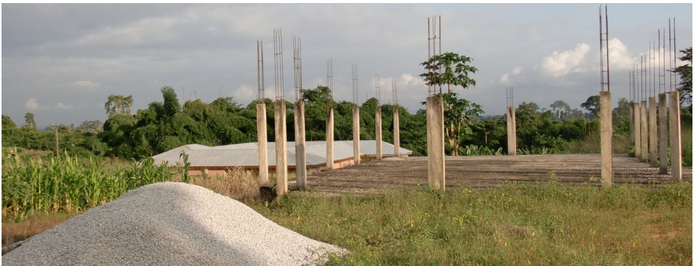
FIGURE 5.7: Unfinished assembly building, five years after construction began
