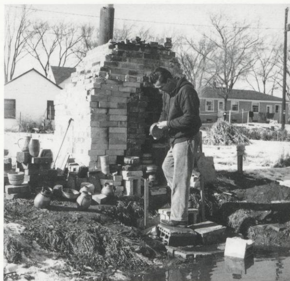
Fig. 6. The salt-fired kiln at Verona, Wisconsin, 1961. Built alongside a drainage ditch, the kiln was flooded unexpectedly during a firing. The steam produced a curious meaty texture and inspired Reitz to try introducing salt as a brine.
