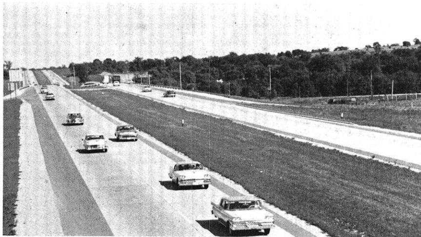
Below: Completed portion of the same highway.
