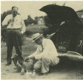
Field testing — measuring stream conditions like dissolved oxygen content by the streambank was a new idea. DNR photo
