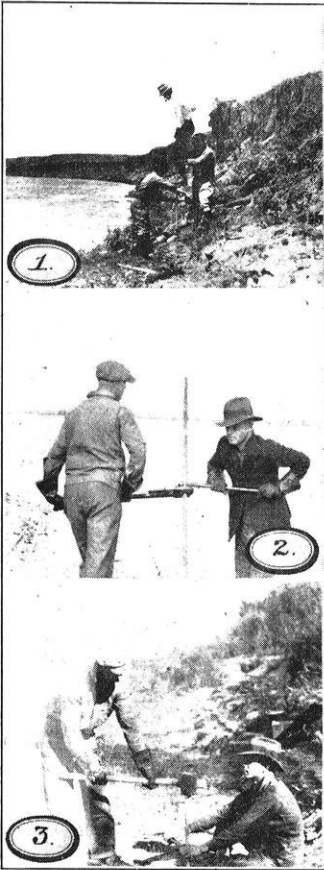
FORCING DOWN DRILL RODS Fig. 1—By Weighting and Turning. Fig. 2—By Turning. Fig. 3—By Driving and Turning.
