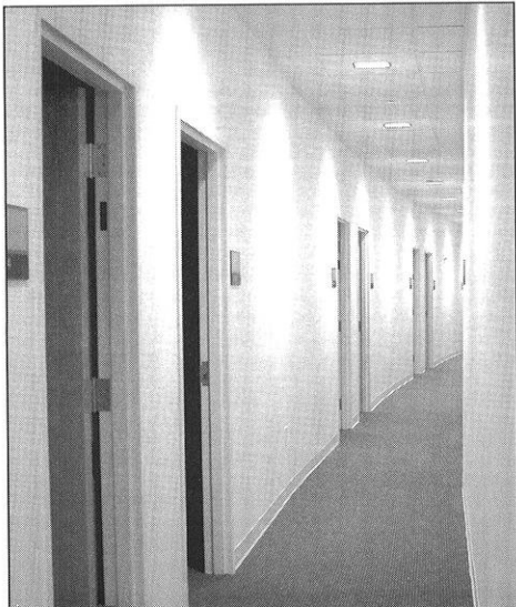
The hallways on the north end of the building are curved.
