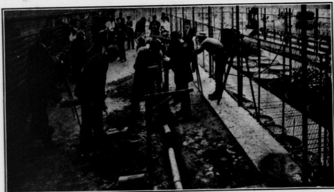
Short Course students are given thorough training in the location and laying of tile drains since such drainage is needed by over 2,000,000 acres of Wisconsin lands.
