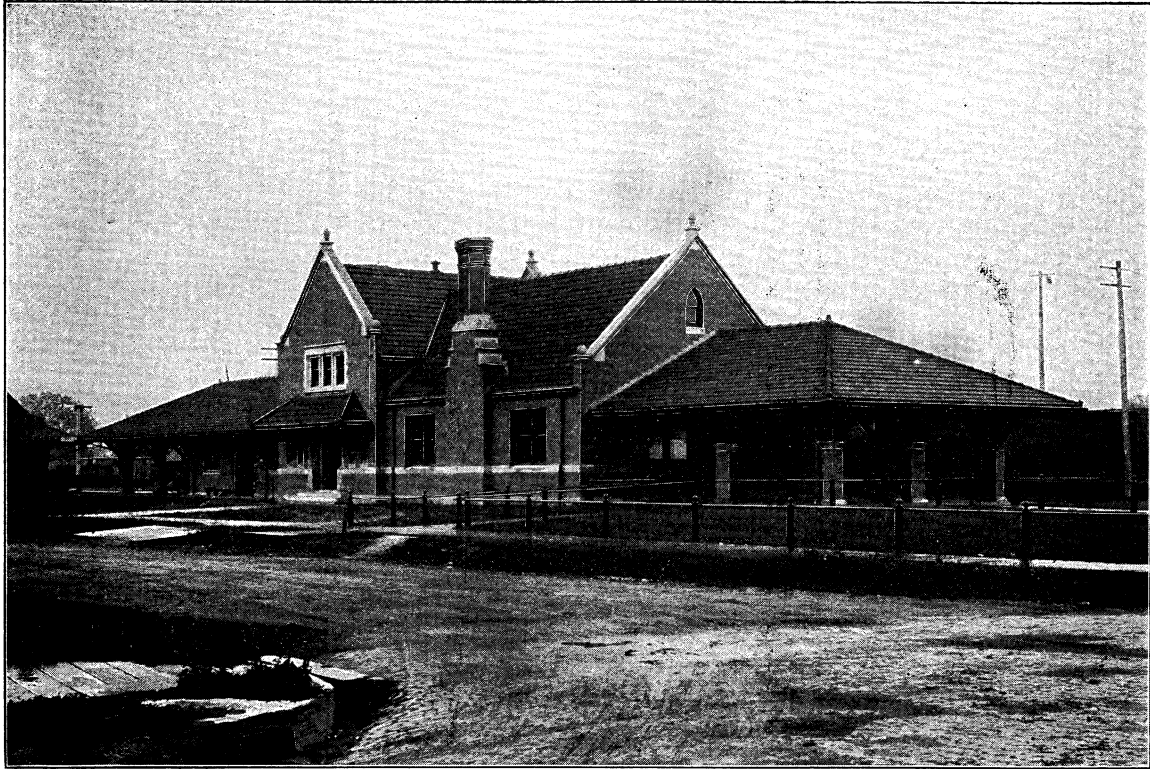
CHICAGO, MILWAUKEE & ST. PAUL RAILWAY.—DEPOT, BELOIT,
