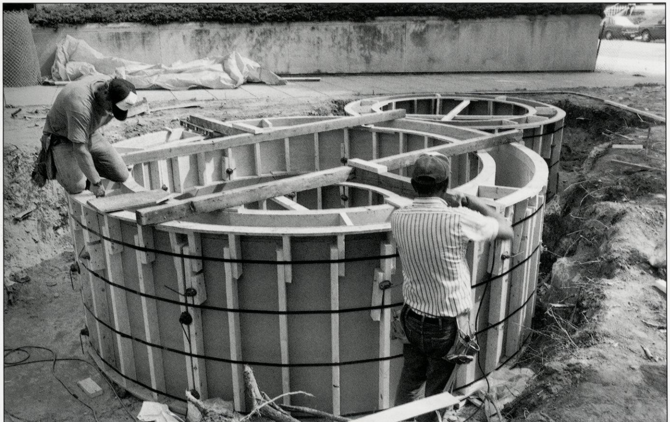
ABOVE: Placing the basic wood and cardboard form for the concrete footing of the sculpture in the east section BELOW: Completing assemblage of form in east section after its height was extended by three inches
