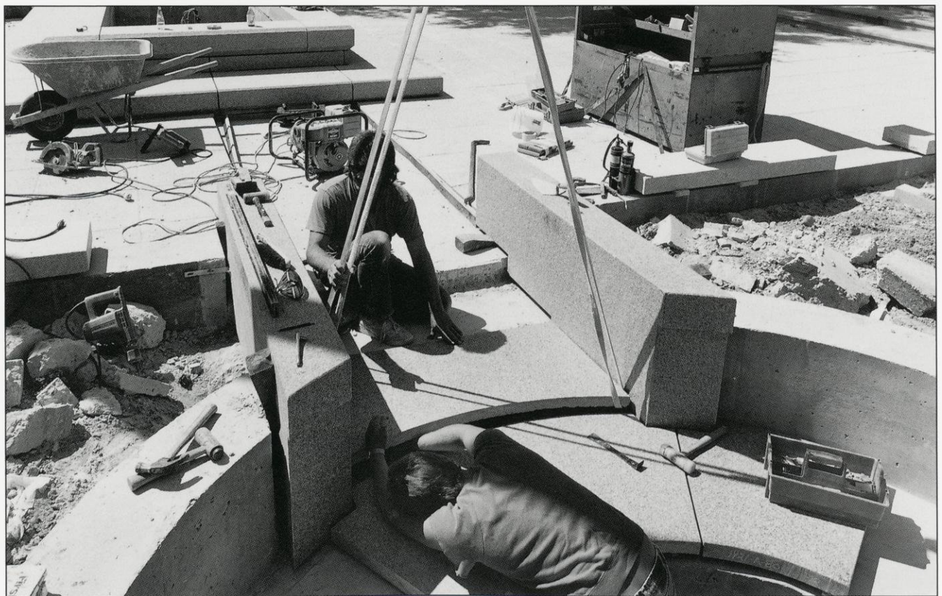
ABOVE: Workmen pouring and scoring the concrete for the central walkway BELOW: Installing granite on top of the concrete base in the east section
