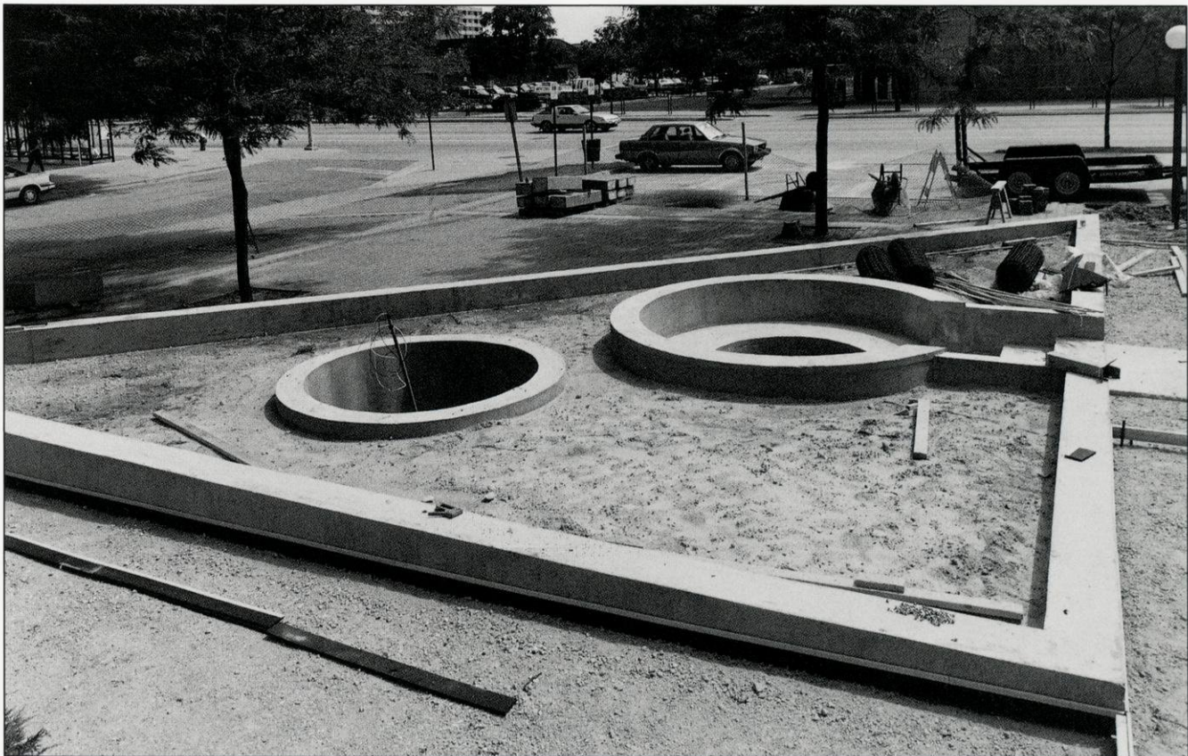
ABOVE: Assembling the forms for the concrete triangle shape in the east section BELOW: The completed concrete footings for the east section
