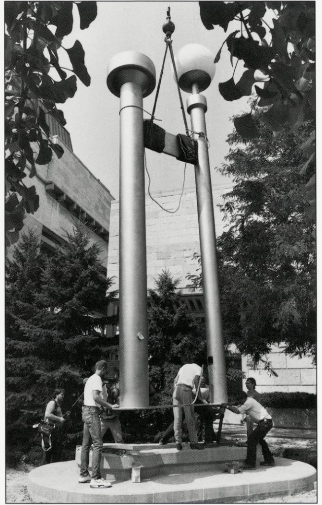
Installing the steel columns in the west and highest section
