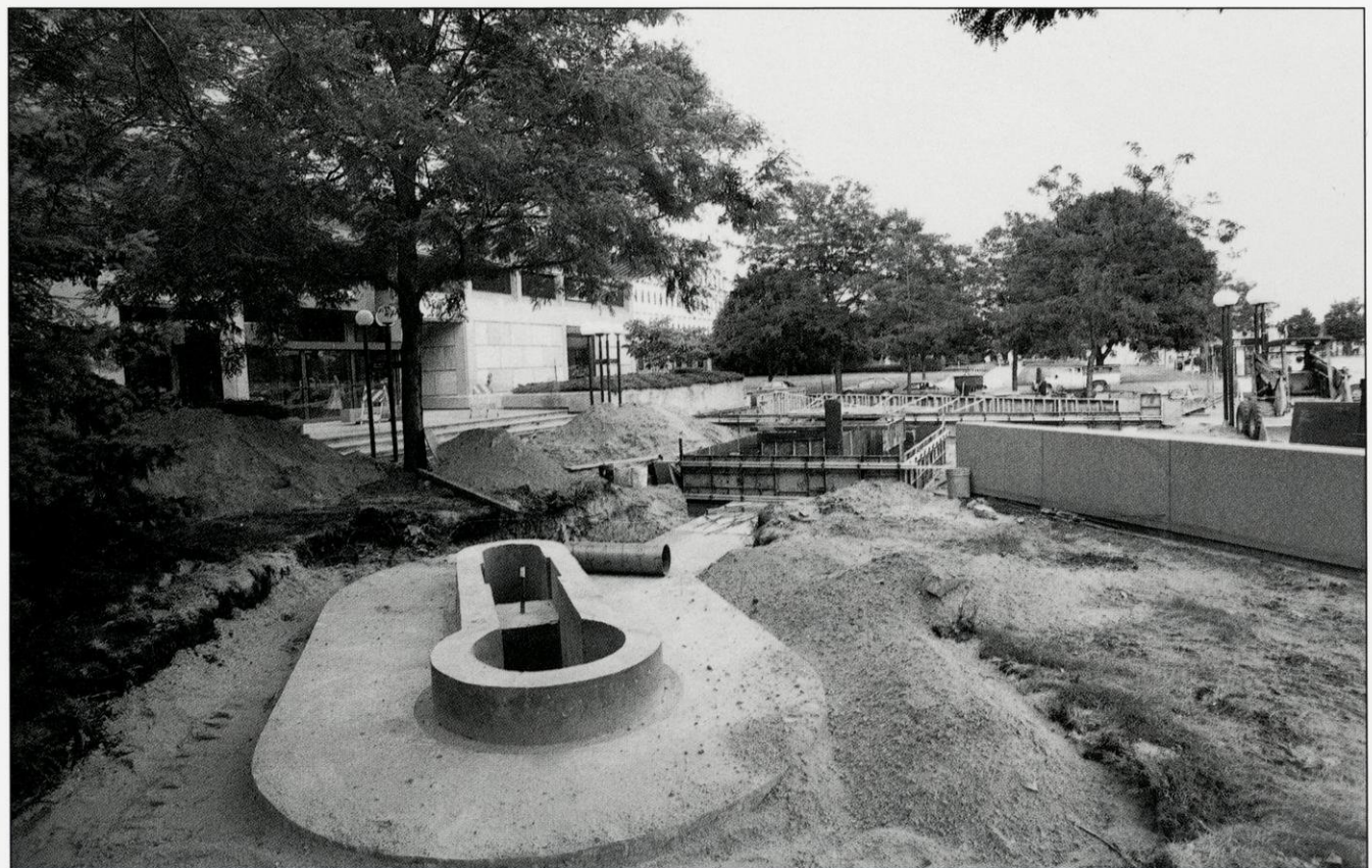
ABOVE: Preparing a level base for the footings in the central section BELOW: Overview of the footings from west to east, with the blp-shaped base in the foreground
