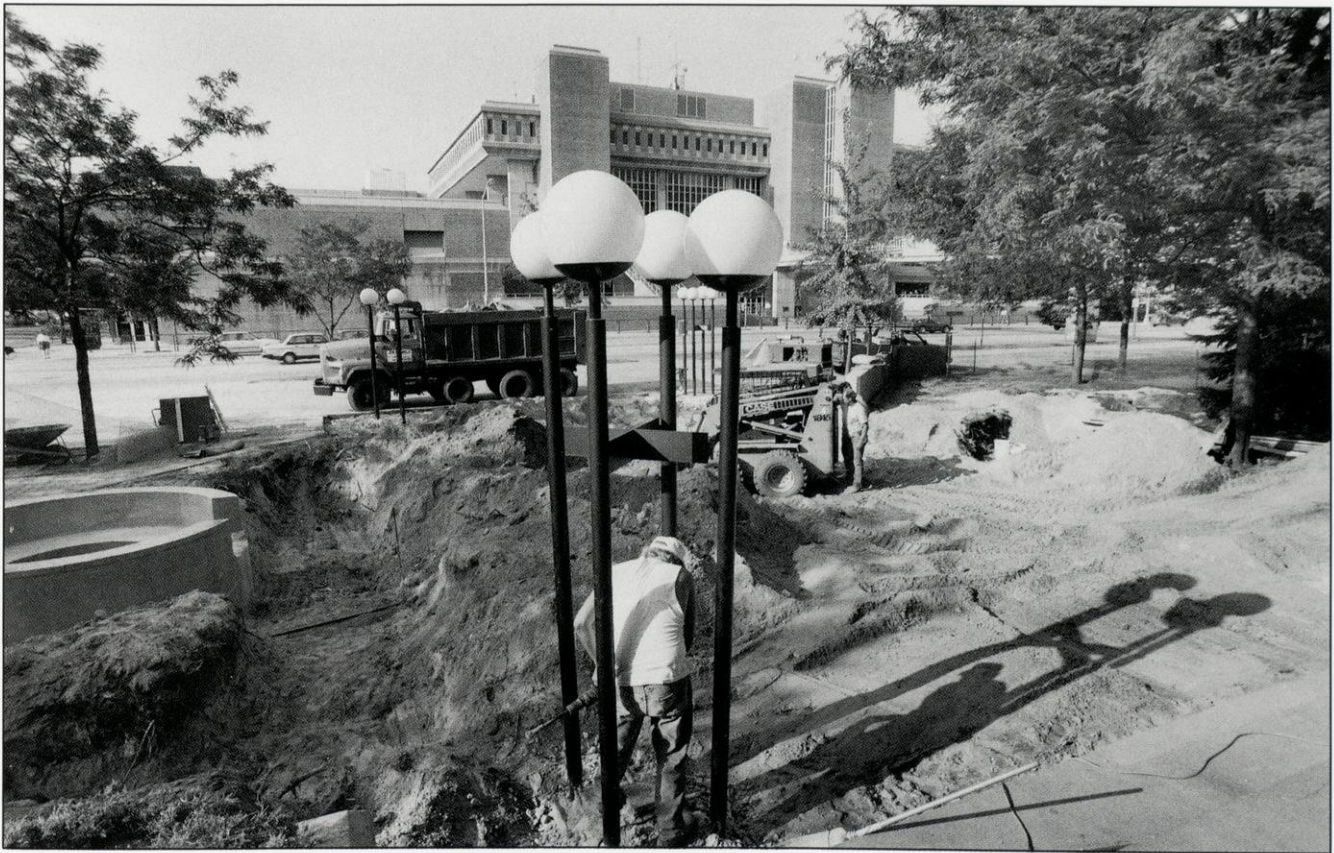
ABOVE: Assembling the form for the blp-shaped base in the east section
