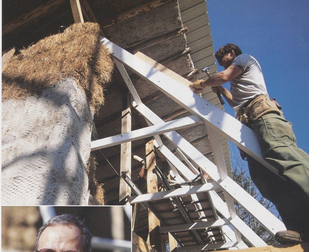
Mark Harrell's home near La Crosse is self-sufficient: it does not rely on utility companies for heat, water or electricity. Plaster-coated straw bales provide both solid structure and excellent insulation.
