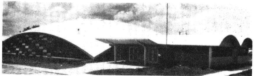
Sections of a sphere and two cylinders form the roof pictured above.
