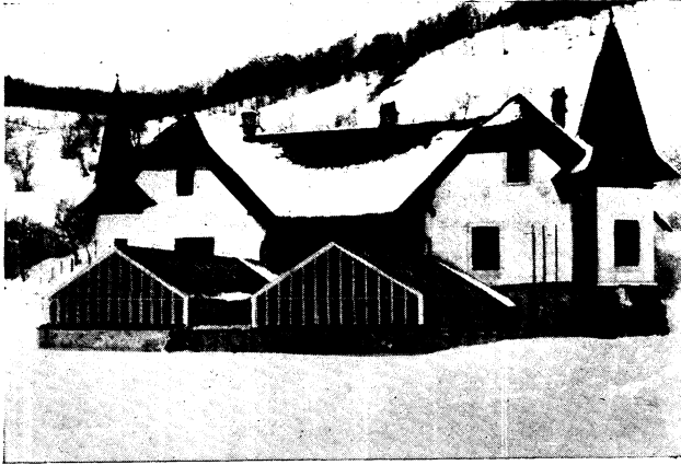
ANNEX OF STATION AT LUNZ, AUSTRIA
