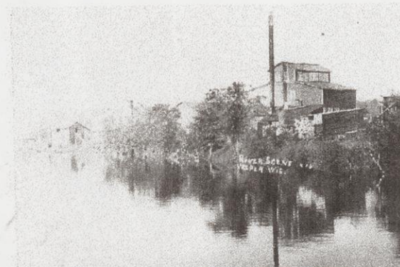
The Silo Factory on the Hemlock Creek
