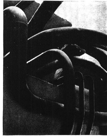
SINUOUS CURVES of welded pipe sweep from floor to floor carrying steam, water, gases and liquids.
