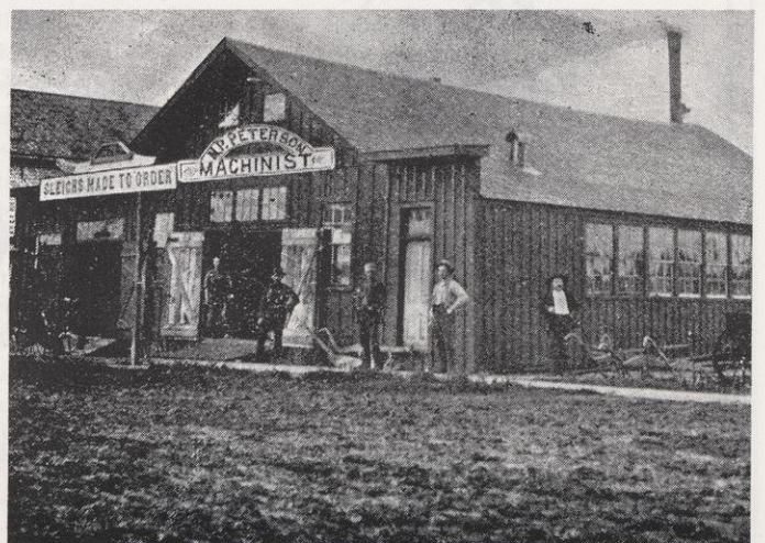
Blacksmith and Wagon Shop of N. P. Peterson
