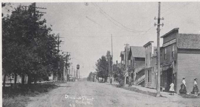
LOOKING NORTH down Division St.—girl on the right is Hildegarde Pribnow by the Pribnow store, formerly the Pradt store. Next is Daines garage, then Schallers Saloon, 1912.
