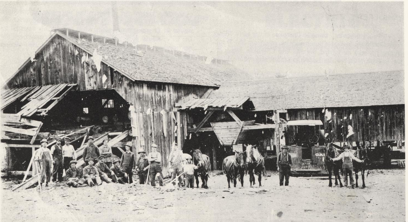
Saw Mill on the west bank of the Eau Pleine river on Highway N owned by Charles Taylor in 1873; by Paul Umhoefer in 1891; by E.
