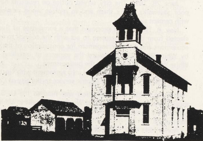
COLBY DISTRICT SCHOOL BUILDING—located across Clark County line in Marathon County, the district in which it was located was a joint district, including portions of the towns of Colby and Hull. Built for two departments. Teachers were Fannie Burton, Laura Gotchy and Carrie Vandercook. The school board were Andrew Flaig, Sam Shafer and R. B. Salter. Both schools were of the same building plan.
