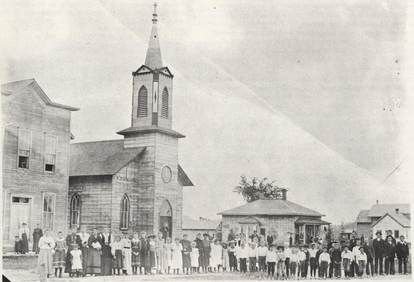
Left to right - - City Hall, before the addition which housed the fire engine. Next, the old St. John's Evangelical Church, built in 1892. This church was destroyed by fire on Feb. 9, 1941. The next building, the residence of Sam Shafer. The small white building is the Phonograph office of Sam and Joel Shafer. Building across from the Phono-
