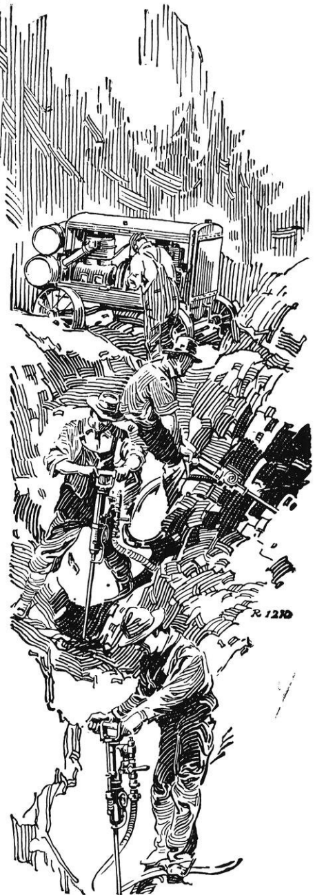
To-day powerful air compressors, both stationary and portable, supply the power for the rock drills
