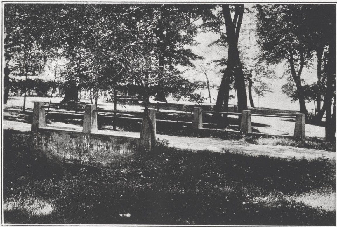
NEW CONCRETE CULVERT WOODWARD'S GROVE
