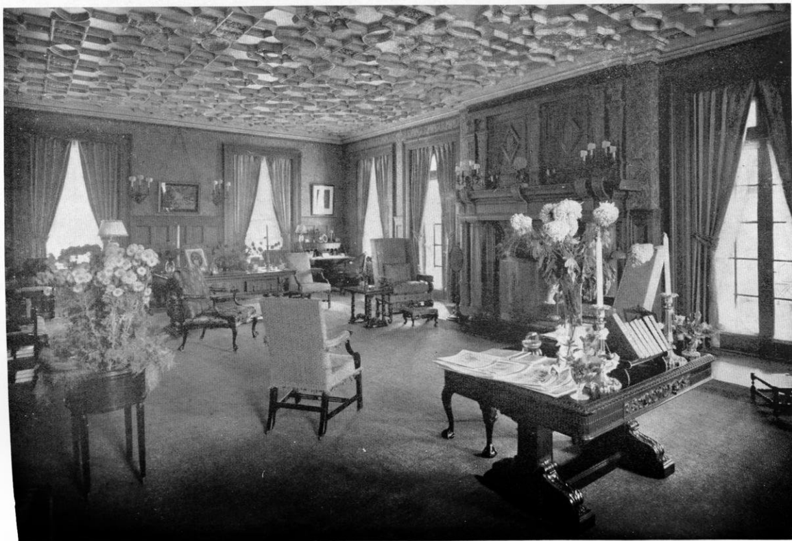
THE LIVING-ROOM IN THE C. W. HARKNESS HOUSE AT MORRISTOWN, NEW JERSEY
