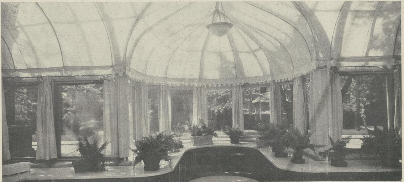
The plant tables are marble-topped and the heating pipes placed underneath, out of sight, behind bronze grilles.
