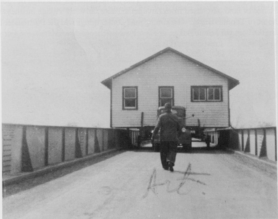
Cottage from Weigands Bay that was moved across the second Prairie du Sac bridge. It had to be jacked up higher in order to clear the bridge railings. Art Eberhart is backing up directing Jack who is driving the truck. Photo taken in 1942.
