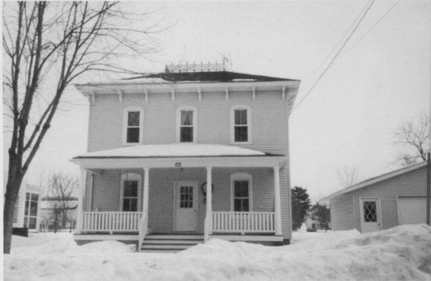
350 Fourth Street: Built in 1912 by John Litscher, this later became the home of Peter Enge, a retired farmer from Honey Creek. It still has the beautiful iron railing on the top.
