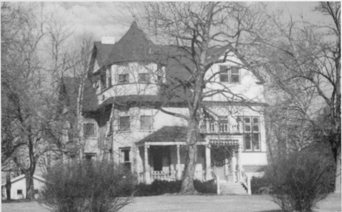
295 Water Street: “.. a proud house high above the river...” – August Derleth . Built in 1889 for Miles Keysar who had moved here from New Hampshire. He was a leader in the growth and development of the village. He was in business and lumber, built the Keysar Grain Elevator, partly owned the Ellen Hardy Steamboat and helped bring in the railroad. The home was designed by Louis Clas, formerly of Sauk City. In addition to the usual rooms the home boasted a library, conservatory, art room and a massive open stairway built of swamp oak. Gumwood, mahogany, rosewood, cherry and walnut were used in addition to red and white oak. Louis Pohlman did the carpentry and Wm. F. Steuber the masonry.
