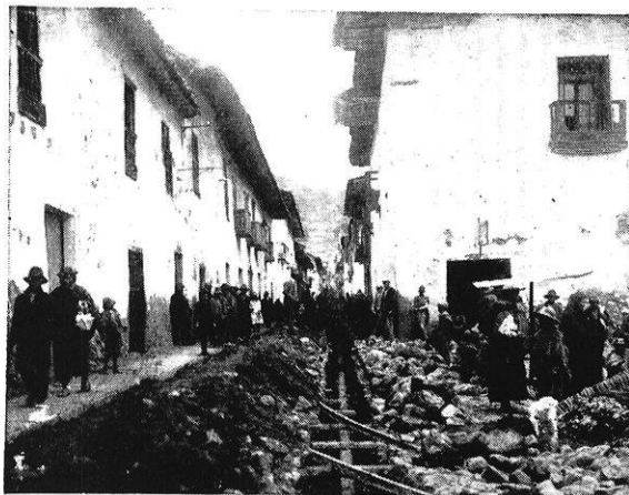
WATER PIPES BEING LAID BY THE FOUNDATION COMPANY FOR THE MUNICIPALITY OF CUZCO, PERU
