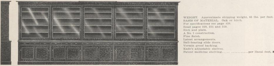
BASIS OF MATERIAL. Oak or birch. For specifications see page 430. Read pages 320, 321 and 329. Rich and plain. A No. 1 construction. Fine finish. Latest arrangements. Ball-bearing slide doors. Vermin proof backing. Kade's adjustable shelves. Patent medicine shelving..... per lineal foot, \$12.75
