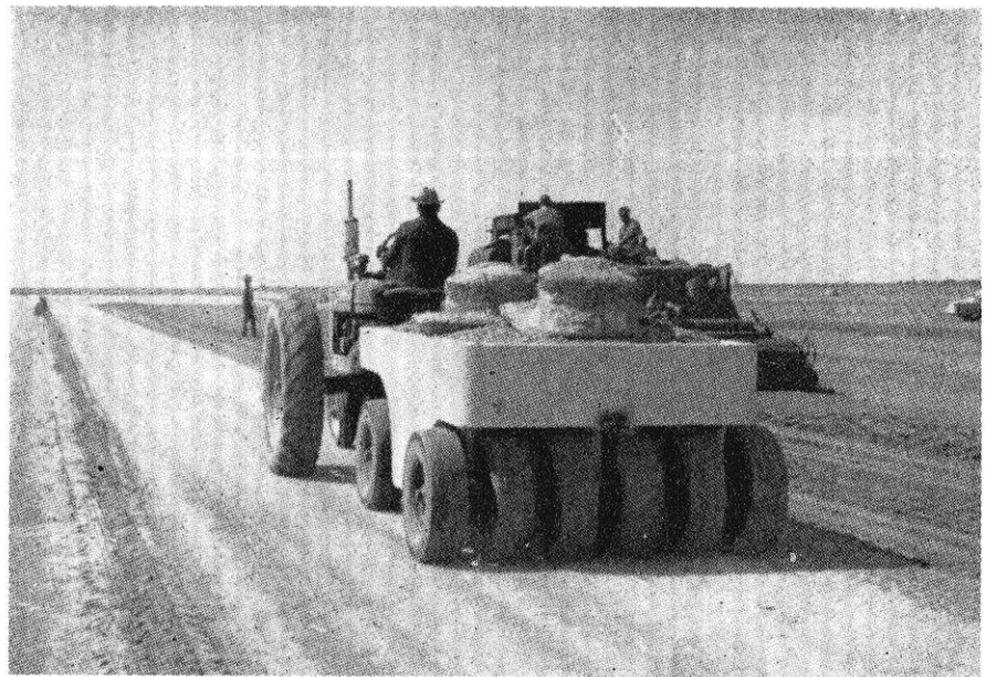
Fig. 12—Pneumatic-tired roller (from PCA)
