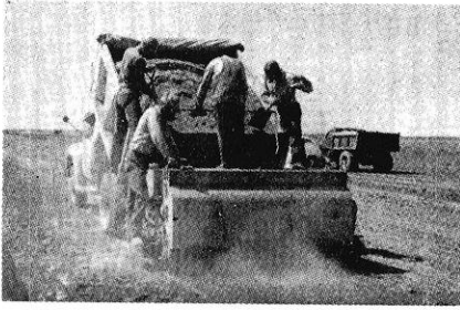
Fig. 7—Mechanical spreader for bulk cement (from PCA)
