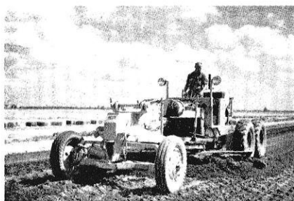
Fig. 4—Grading a runway to crown and grade after pulverization (from PCA)
