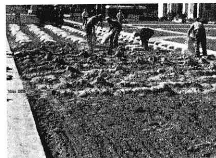
Fig. 5—Spreading cement in bags by hand (from PCA)
