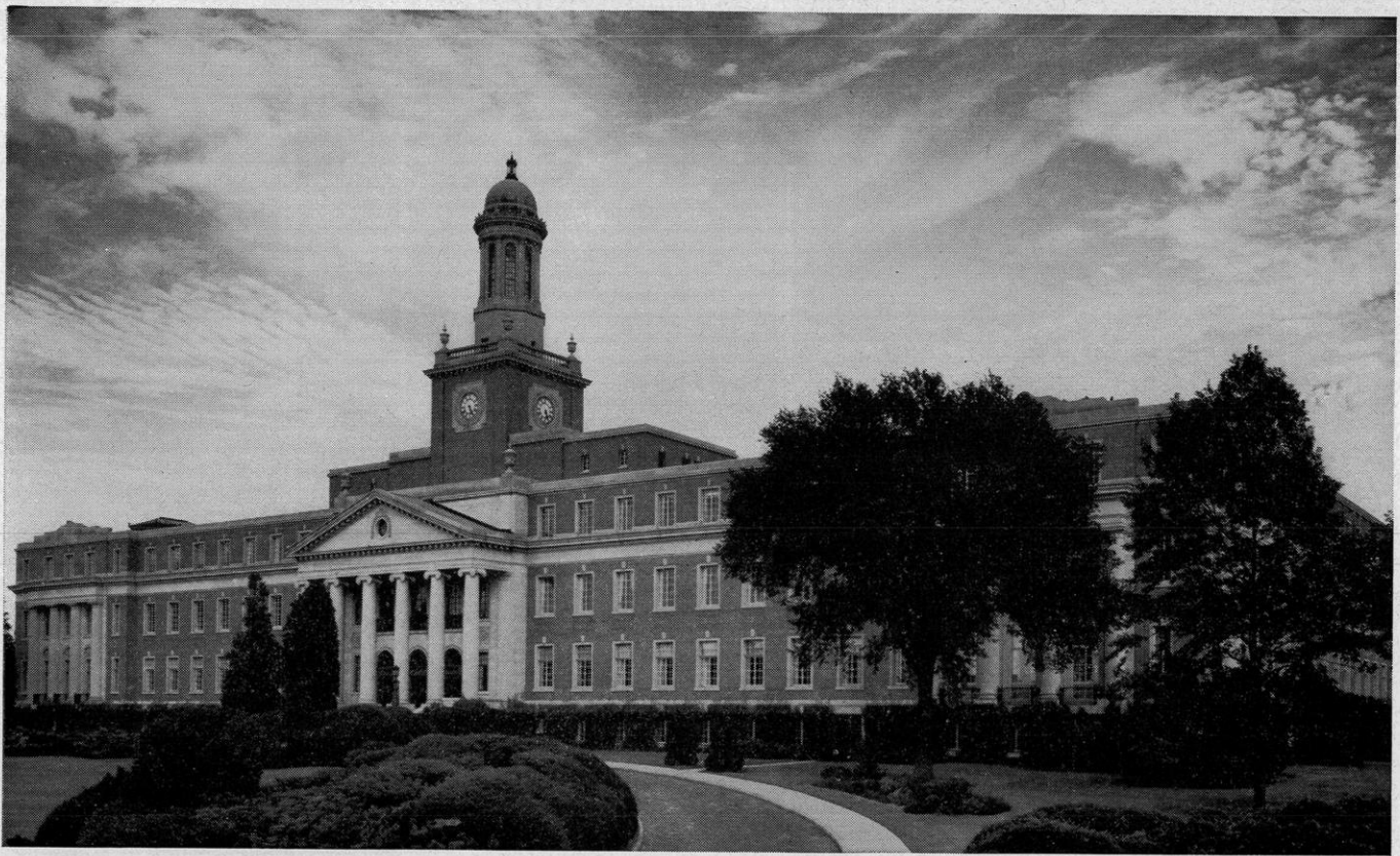
Massachusetts Mutual Home Office
