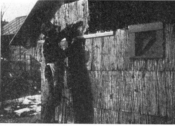
NAILING BARK ON A ROUGH BOARD SIDING COVERED WITH TAR FELT.
