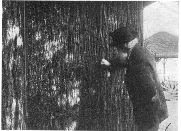
JOHN BURROUGHS INSPECTING CHESTNUT BARK THAT HAS BEEN ON THE BUILDING TWENTY-FIVE YEARS.
