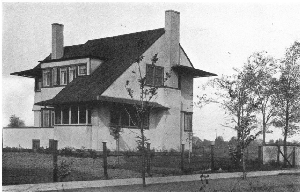
CEMENT HOUSE WITH GOOD ROOF LINES AND MOST UNUSUAL AND INTERESTING ARRANGEMENT OF GROUPS OF WINDOWS: A DESIGN ESPECIALLY SUITED TO LOW-LYING COUNTRY. A TYPE OF WESTERN CEMENT ARCHITECTURE, INTENDED FOR A NARROW PLOT IN TOWN OR VILLAGE.
