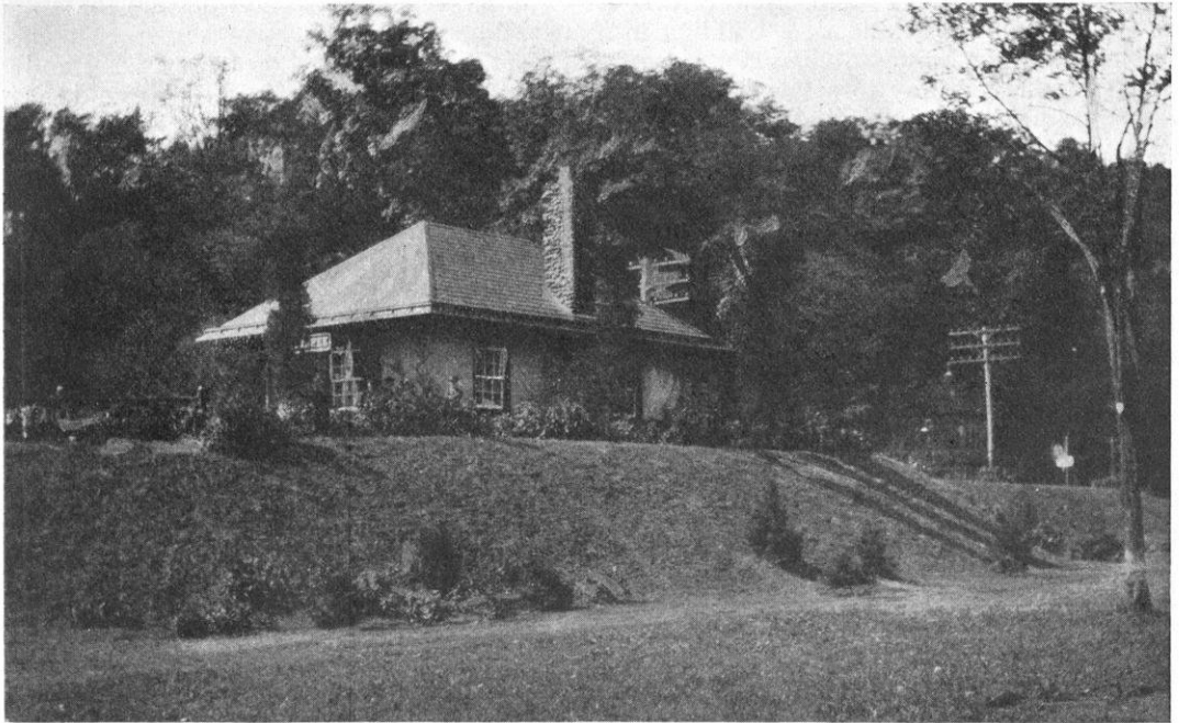
MOUNTAIN STATION ON THE PENNSYLVANIA RAILROAD SHOWING A JUST COMPLETED NATURALISTIC PLANTING, MOST OF THE SHRUBS AND TREES HAVING BEEN TRANSPLANTED FROM THE WOODS IN THE NEIGHBORHOOD: THIS IS ONLY ONE OF MANY EXAMPLES OF HARMONIOUS TREATMENT OF BUILDING AND GROUNDS.
