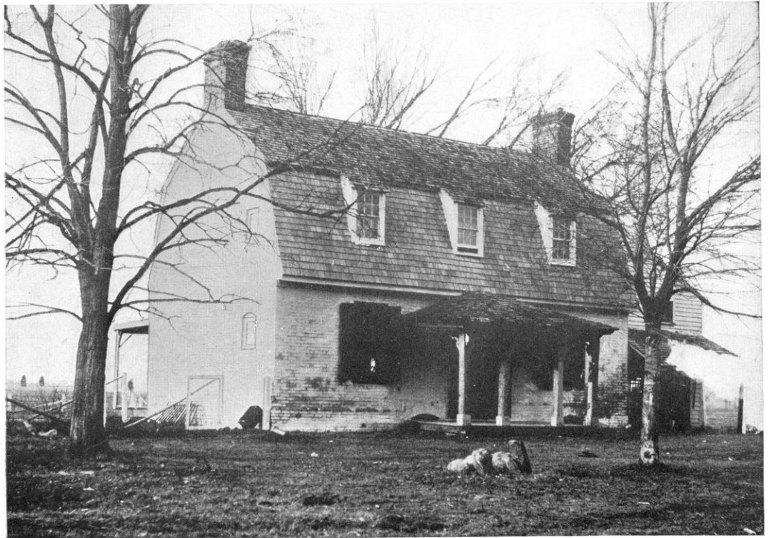
FIGURE 4-A: TWO VIEWS OF ANOTHER INTERESTING EXAMPLE OF THE SOUTHERN COTTAGE WITH GAMBREL ROOF: THESE PHOTOGRAPHS ARE FROM AN EIGHTEENTH CENTURY HOUSE AT DOVEY BRIDGE, MARYLAND: ON THE NEXT PAGE IS SHOWN MR. BRINCKLOE'S DEVELOPMENT OF THIS RATHER SIMPLE HOME INTO A COMFORTABLE MODERN COTTAGE WITH GOOD-SIZED LIVING ROOM, DINING ROOM, FOUR BEDROOMS AND A SPACIOUS BATH: FLOOR PLANS TO BE FOUND ON PAGES 119 AND 120.
