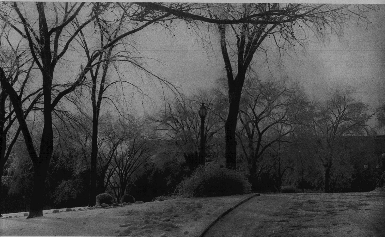
A FEBRUARY SNOW BLANKETS THE HILL AND SOFTENS THE LINES OF THE BIOLOGY BUILDING
