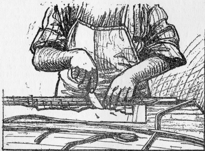
FITTING LEAD IN AROUND THE GLASS.
