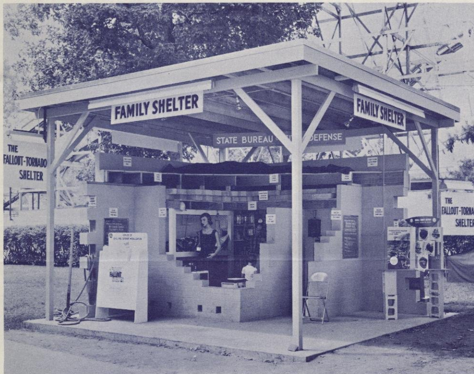
MODEL BASEMENT FALLOUT SHELTER AT FAIR GROUNDS
