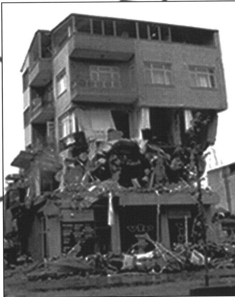
Scenes like this from the 1999 Turkey earthquake have given researchers more incentive than ever to develop better earthquake-resistant structures.
