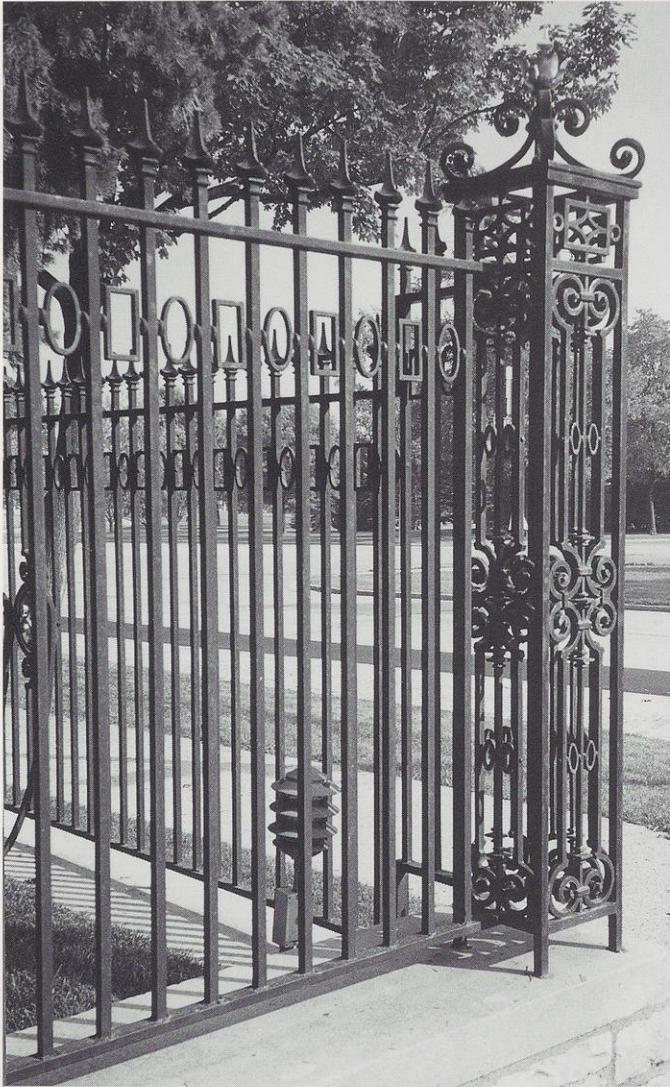
ABOVE: Fence detail, Newberry Boulevard, Milwaukee. Colnik softened the squared rails and simple geometric shapes with a corner box decorated with scrolls, topped with a gold-leafed flower.
