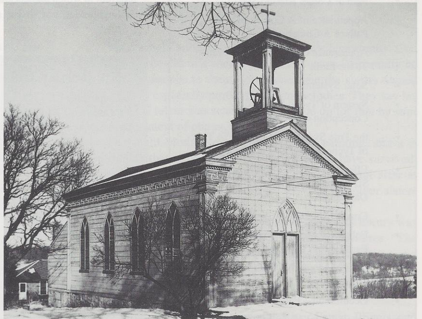
St. Augustine’s Church in New Diggings, one of the masterworks of Wisconsin architecture, designed and built by Mazzuchelli in 1844. The nine-inch planks used for the exterior were tooled to simulate stone, reminiscent of the magnificent Italian churches Mazzuchelli knew in his youth. It is now on the Wisconsin Preservation Trust list of threatened buildings.
