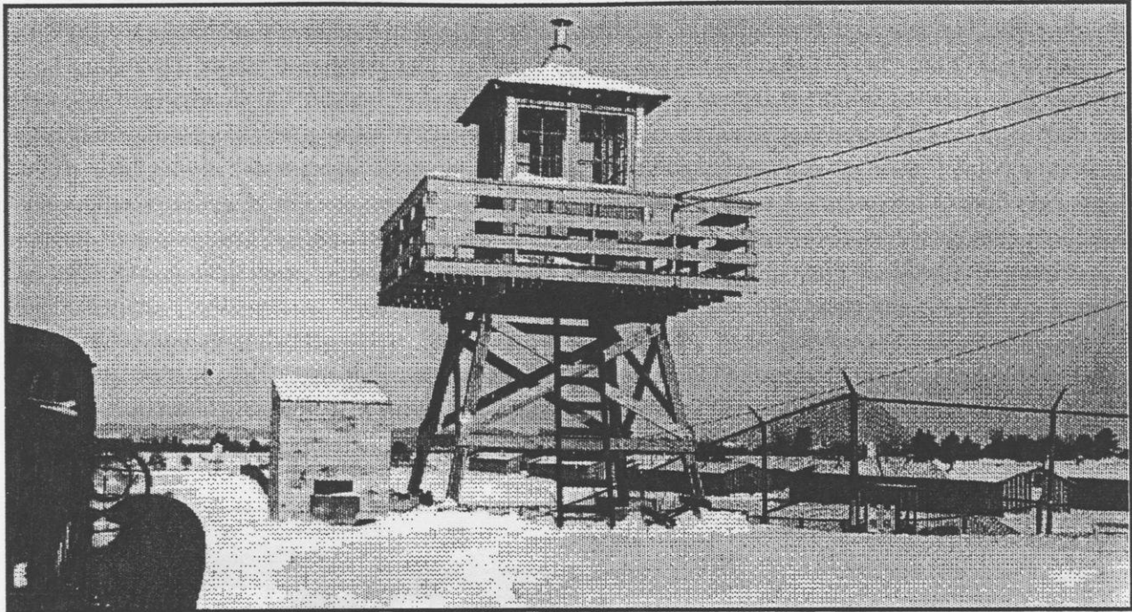
Figure 7. Guard tower, ca. 1942. Guard towers at the internment camp consisted of a small sentry house placed on a "scaffolding" type base. Source: "WWII POW Camp" file.
