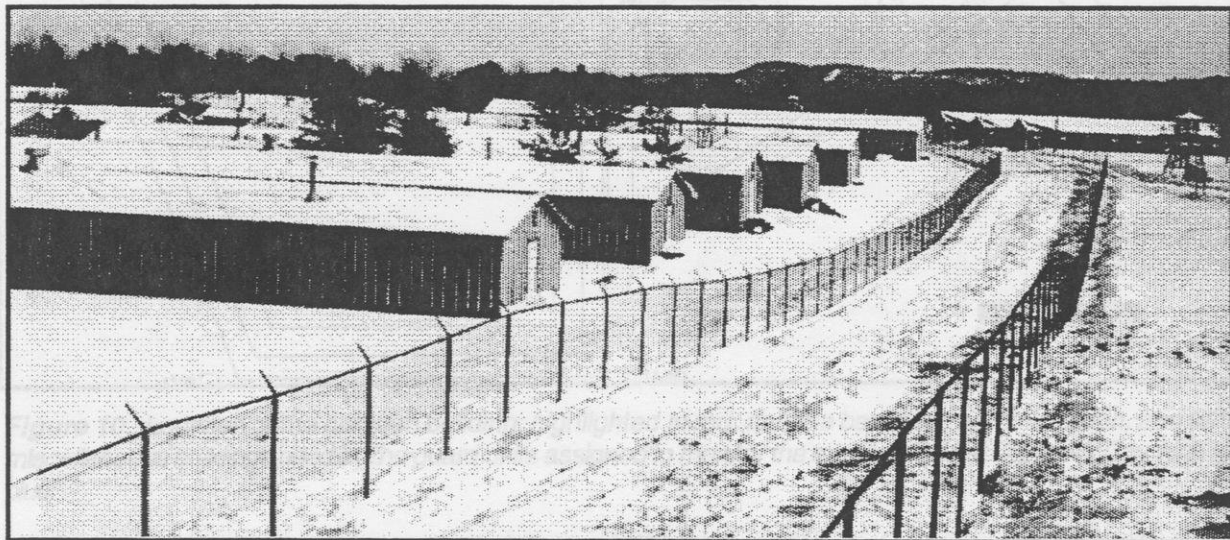
Figure 9. The internment camp barracks were constructed of tar paper and lath walls erected over a rectangular concrete pad. Source: "WWII POW Camp" file.
