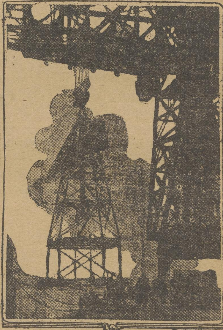
Giant crane lifting a smaller one weighing 310 tons.
